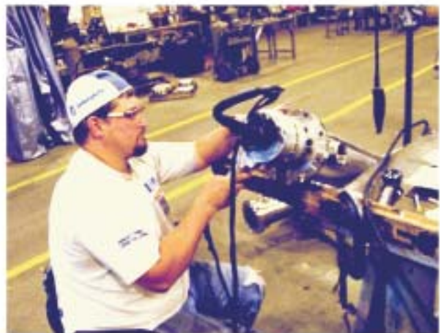
Seal-welding the tubes to the tubesheet
